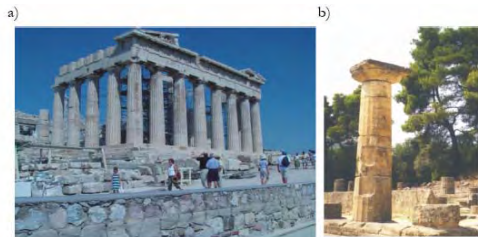
Figure 7.27 Ancient Greek Temple: a) General View and b) Segmental Column
